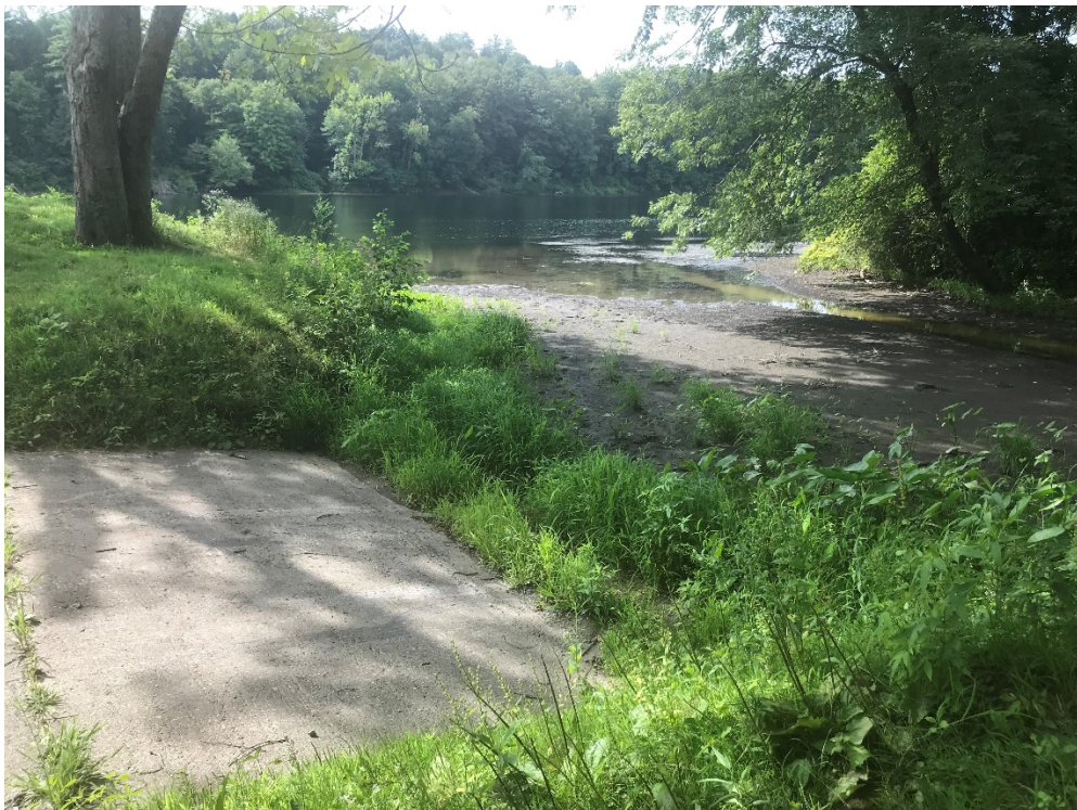
Figure 2. A new ramp (top image) was constructed this past summer at the Dummerston Access Area on the Connecticut River in Dummerston, VT. The old ramp (bottom image) was located in a small back water that had been completely filled with silt and was no longer usable.
